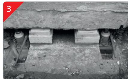
3. Jacks are installed on hardened concrete around the perimeter of the foundation.
