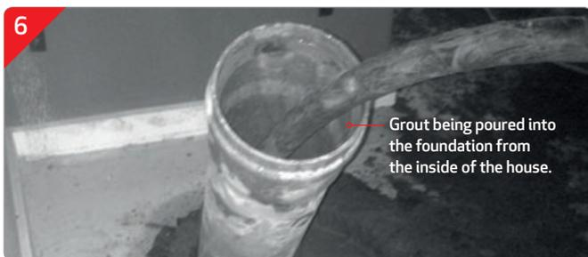
6. Once the house is raised, voids under the foundation are filled with grout.
