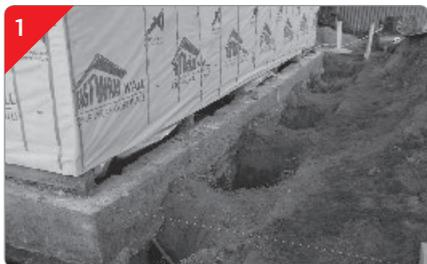
1. Pits are dug out around the perimeter of the foundation at specified spacing and depths.
