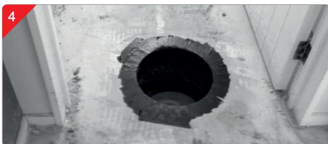
4. Holes are drilled inside the house (at set points) for the concrete floor to be lifted internally in tandem with the perimeter foundation.
