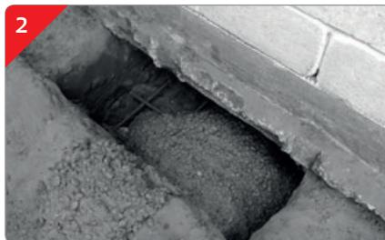
2. Concrete is poured partially into the pits and left to harden, once this has occurred mechanical jacks are placed on top of the concrete.
