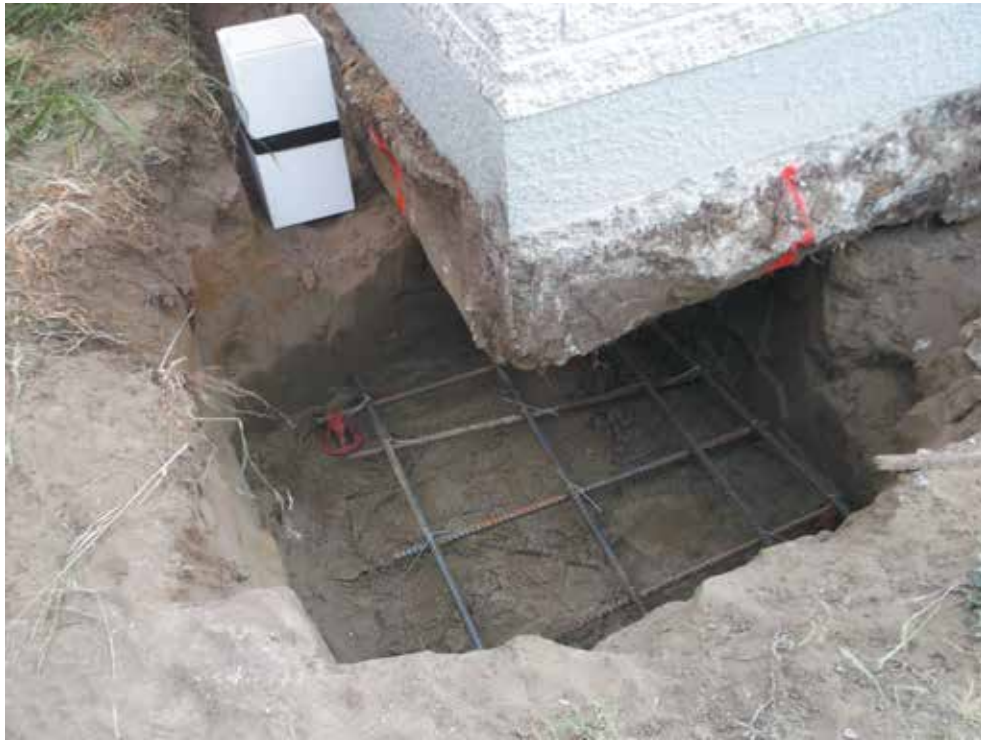
Image 5: Jacking points excavated and reinforcing installed
