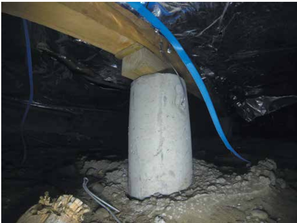
Image 10: H5 timber packers installed, prior to jacks being removed
