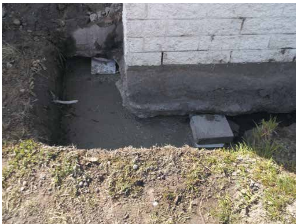
Image 6: Concrete jacking pads poured and polystyrene inserted for reusable jacking voids
