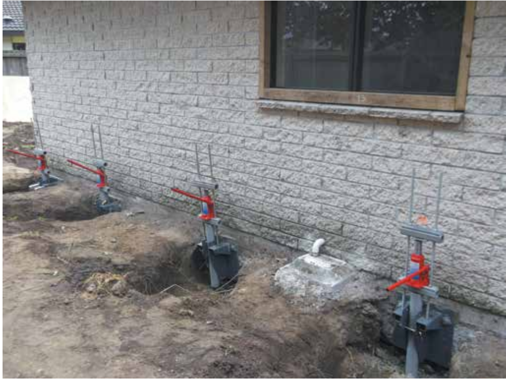
Image 7: Jacks fitted to brackets
