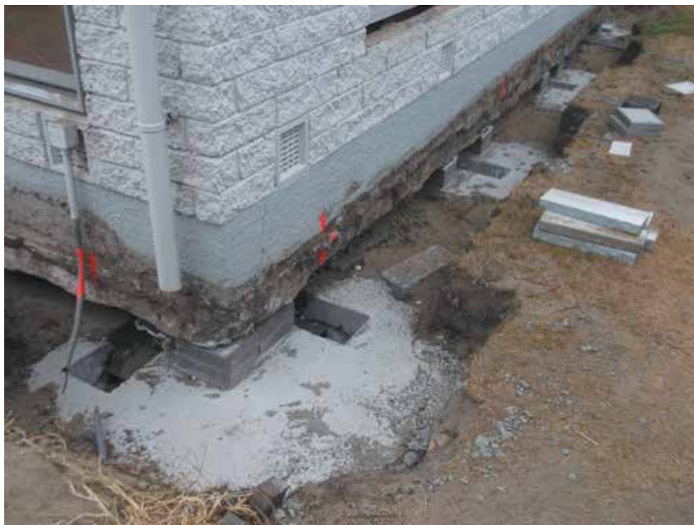
Image 9: Entire foundation packed and jacks removed ready for void fill
