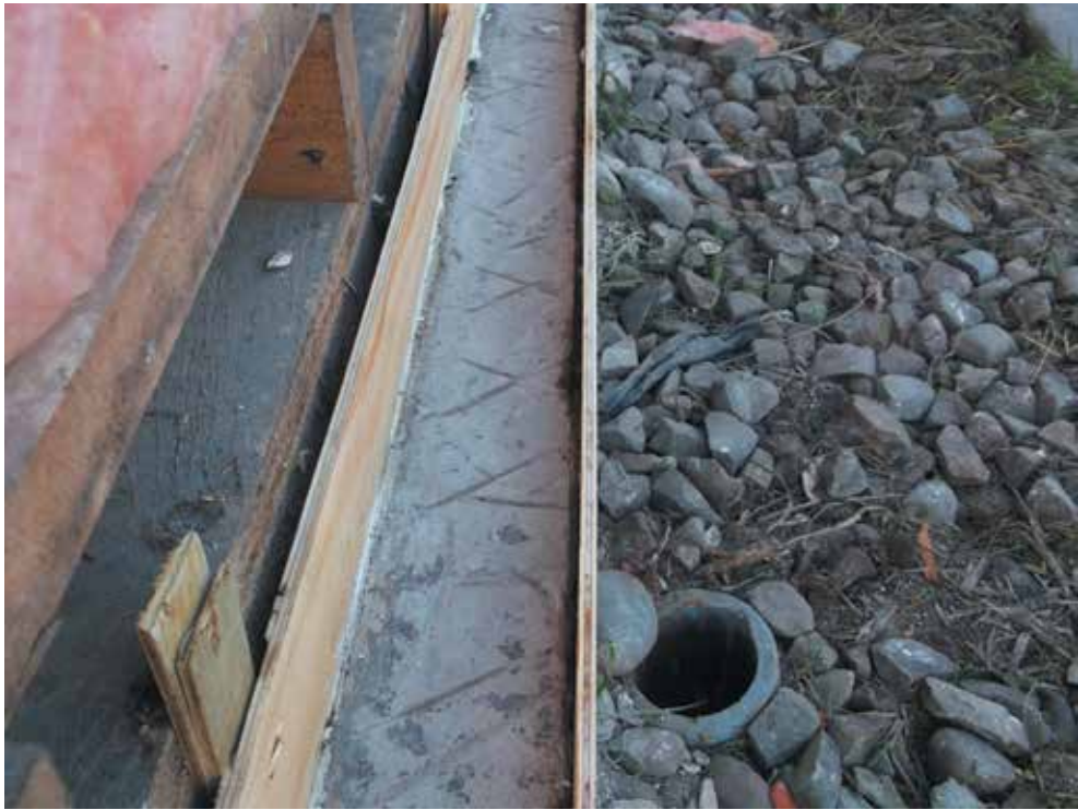
Image 7: Foundation scabbled and formwork ready for topping
