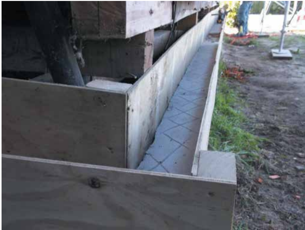
Image 8: Foundation cleaned and scabbled. Formwork installed for pouring of foundation topping
