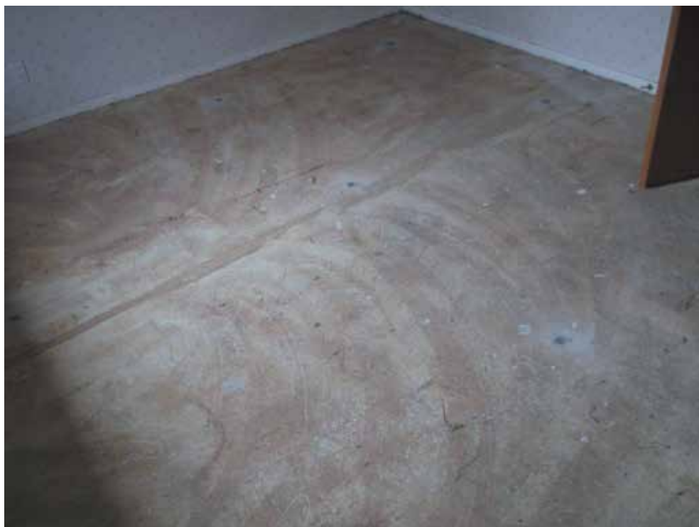
Image 9: Injection points sealed to retain damp proof slab
