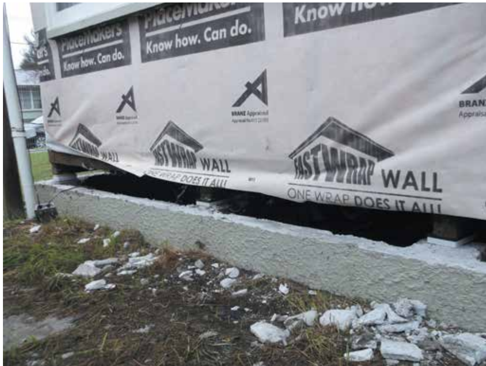
Image 5: Cladding removed, new insulation and wrap installed. Bearers packed
