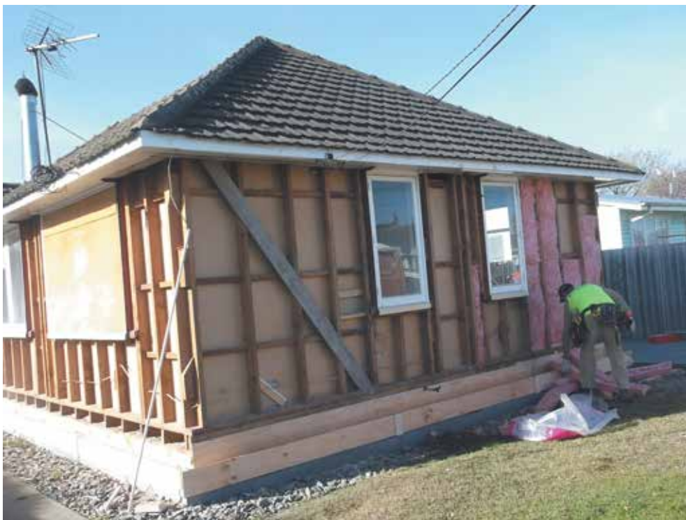
Image 6: Foundation formwork ready for topping. Insulation being installed
