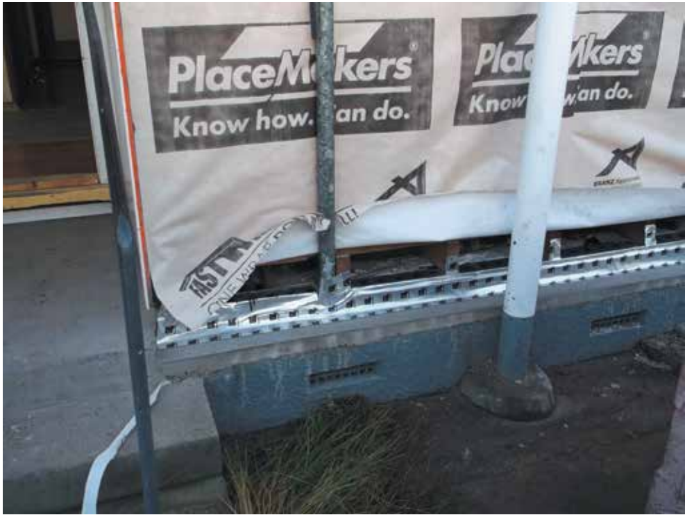
Image 9: Topping poured, flashing tape placed to seal cavity
