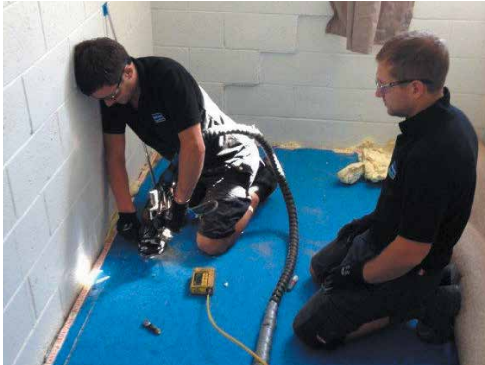
Image 8: Resin injection lifted and filled voids under internal floor slab
