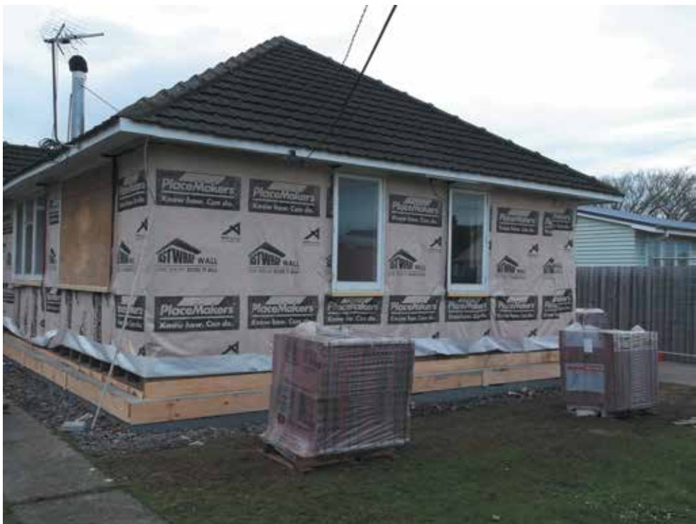
Image 8: Insulation and wrap in place
