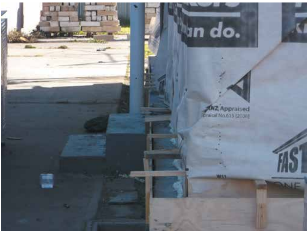
Image 8: Foundation formwork in place
