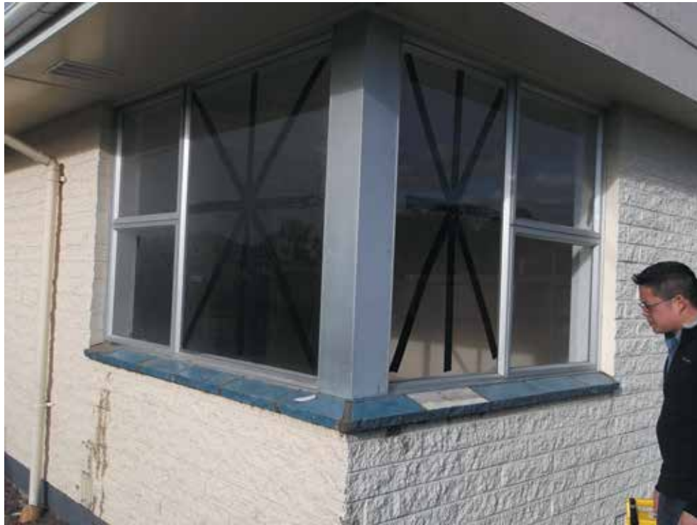
Image 8: Sills and bricks that loosened during jacking and packing reinstated
