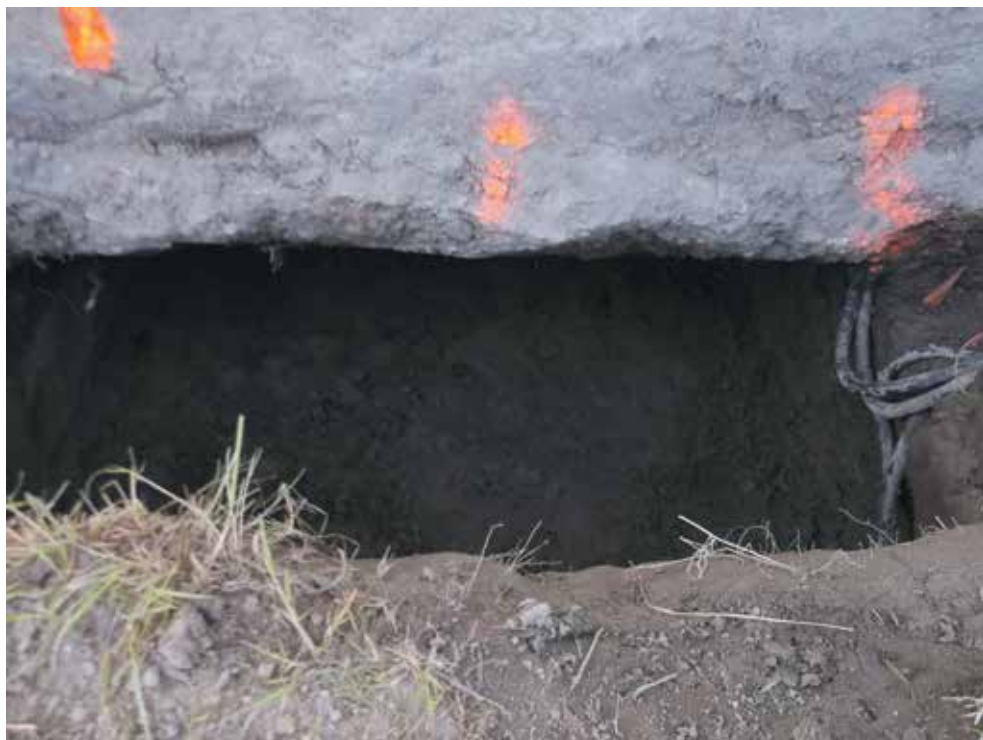
Image 5: Excavated jacking points as per engineer's specifications
