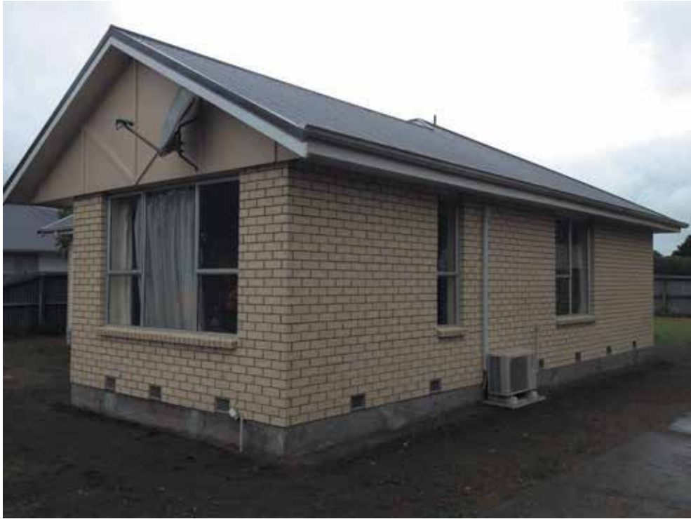
Image 13: Relevelled, reclad and reroofed
