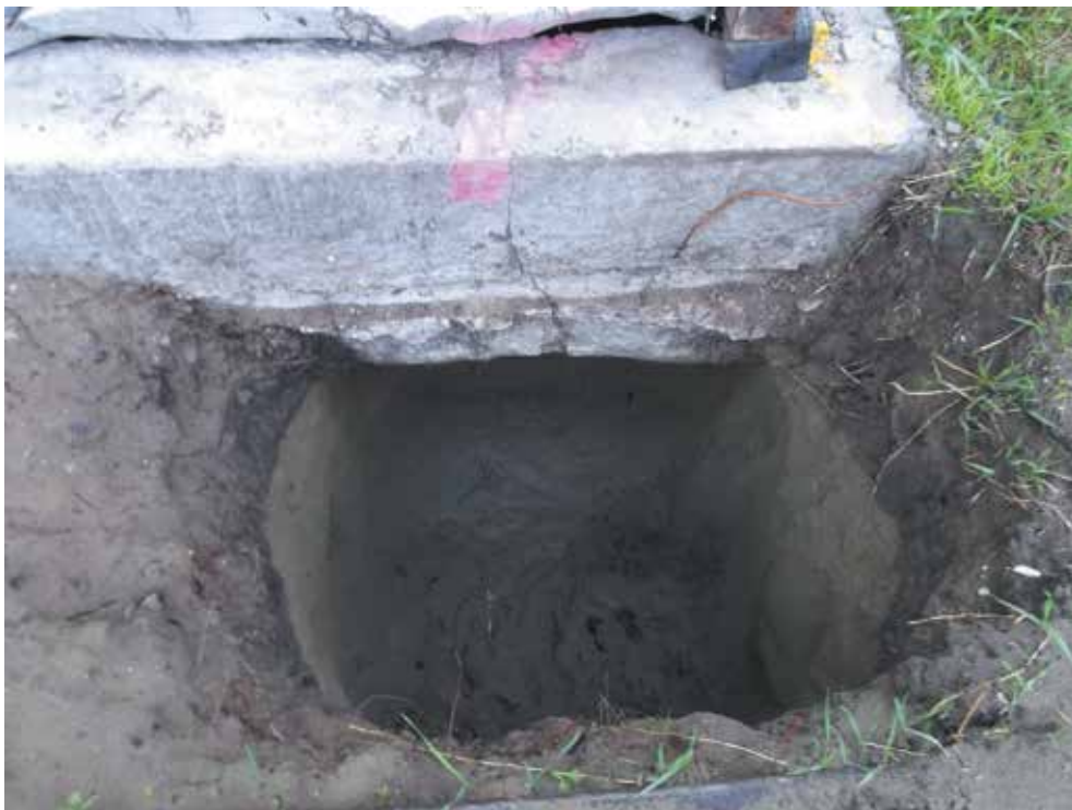
Image 6: Jacking points excavated under foundation cracks as specified by engineer
