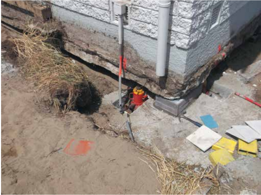
Image 7: Perimeter ring foundation jacked and packed
