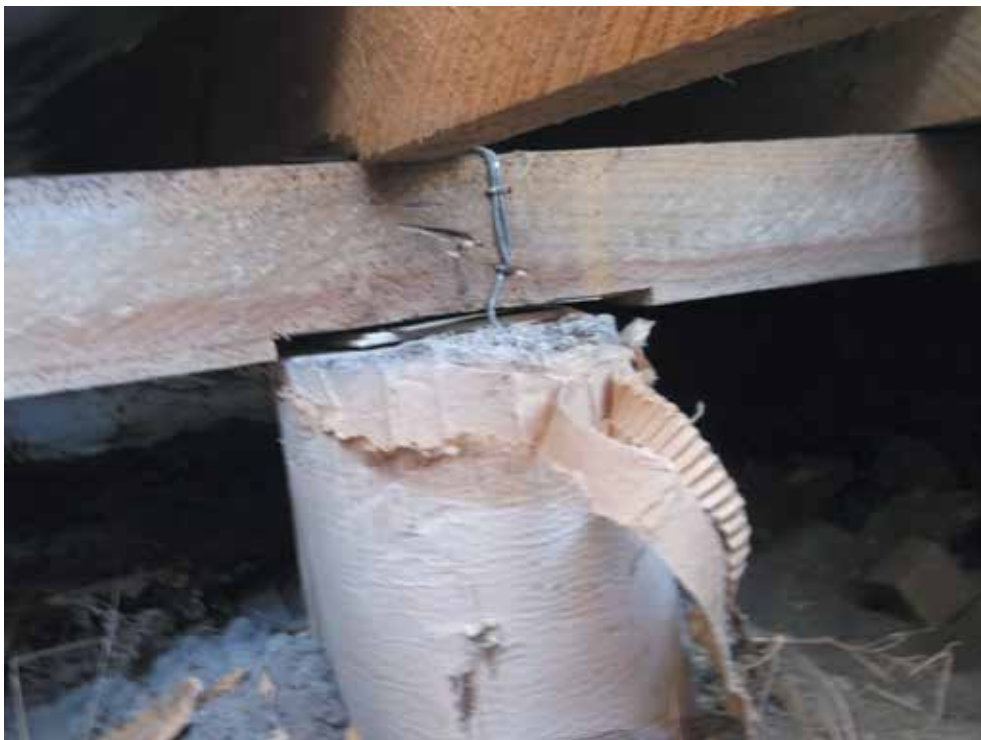
Image 5: Piles packed or notched where necessary to create required level
