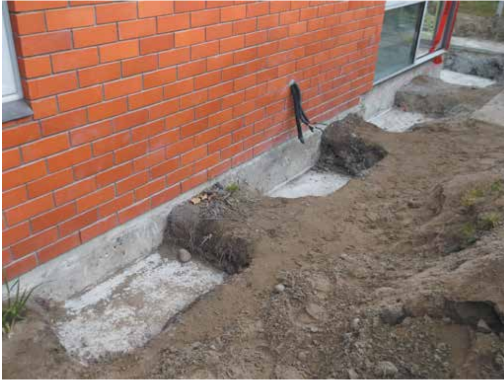
Image 8: Void filled under footing
