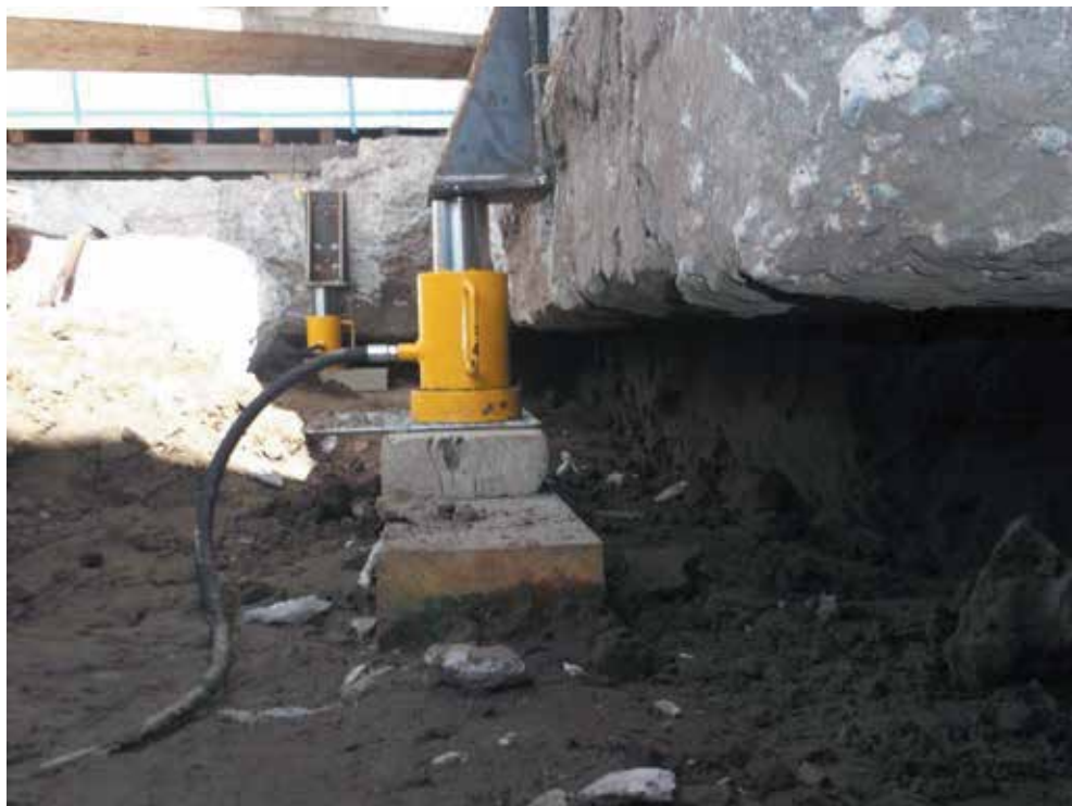
Image 6: Foundations mechanically jacked to required height
