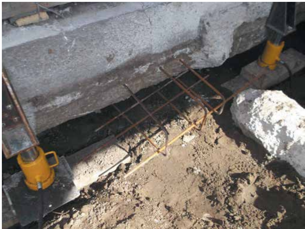
Image 8: Reinforcing installed under foundation cracks as per engineer's specification
