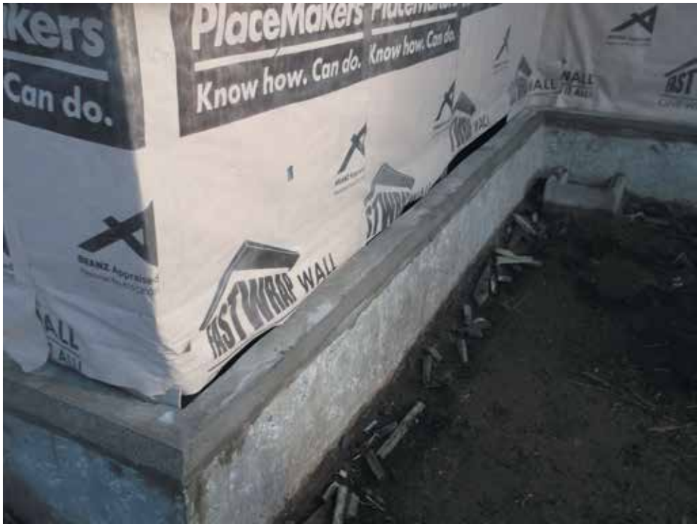
Image 10: Chamfer ground on top of foundation
