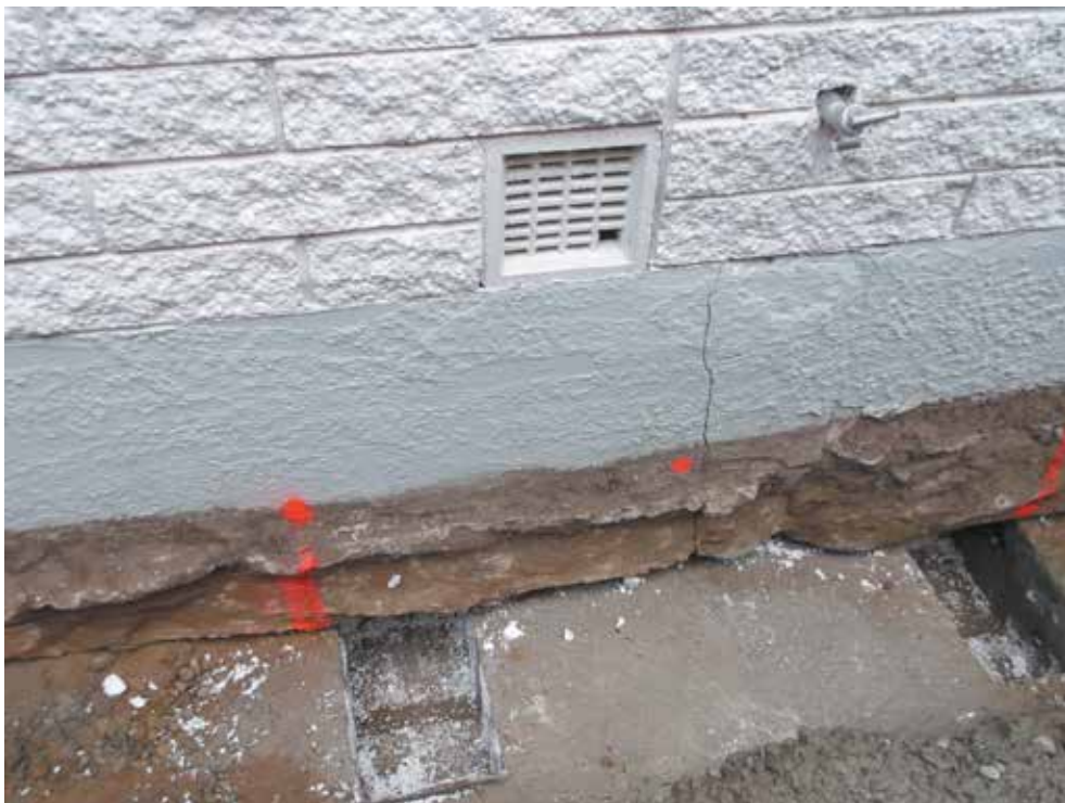
Image 6: Concrete jacking pads poured up to bottom of footing
