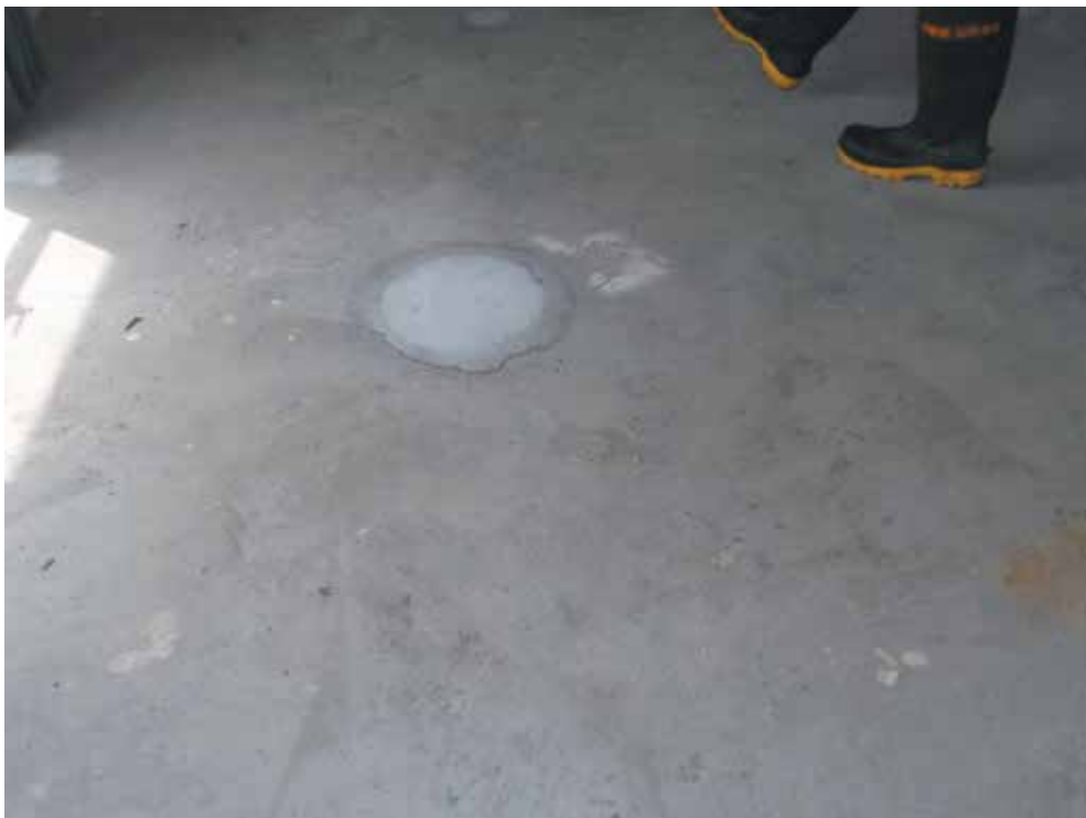
Image 10: DPM reinstated and concrete slab core holes sealed
