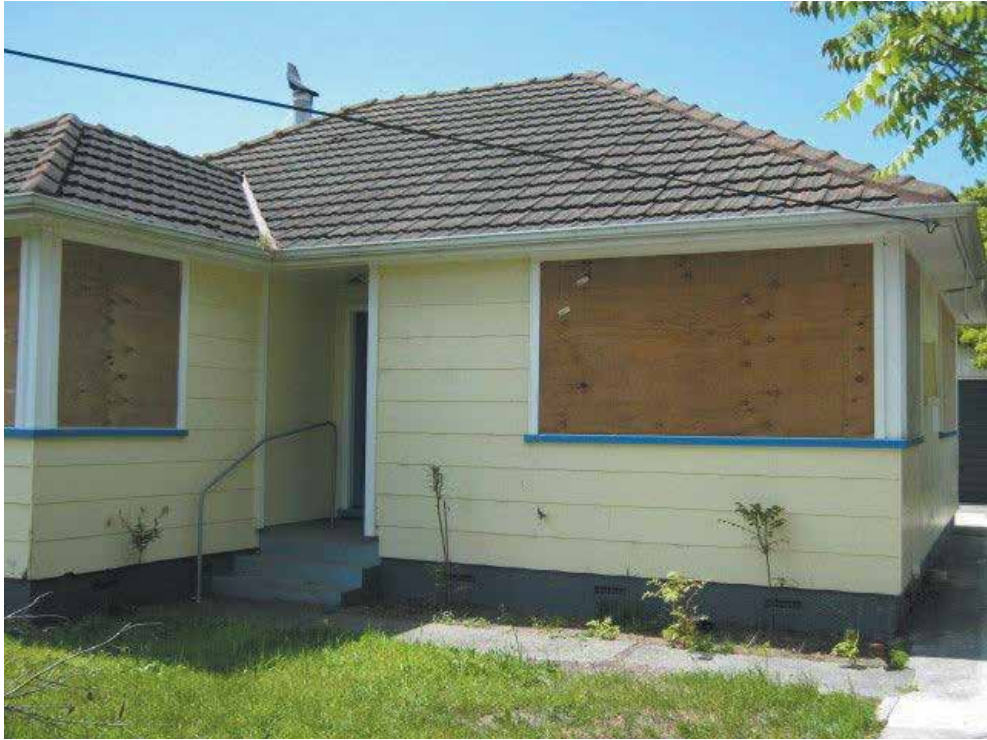
Image 2: No earthquake damage to exterior cladding
