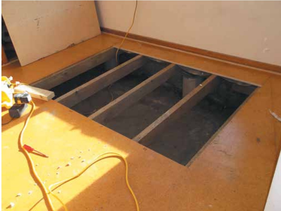
Image 4: Flooring removed to access subfloor
