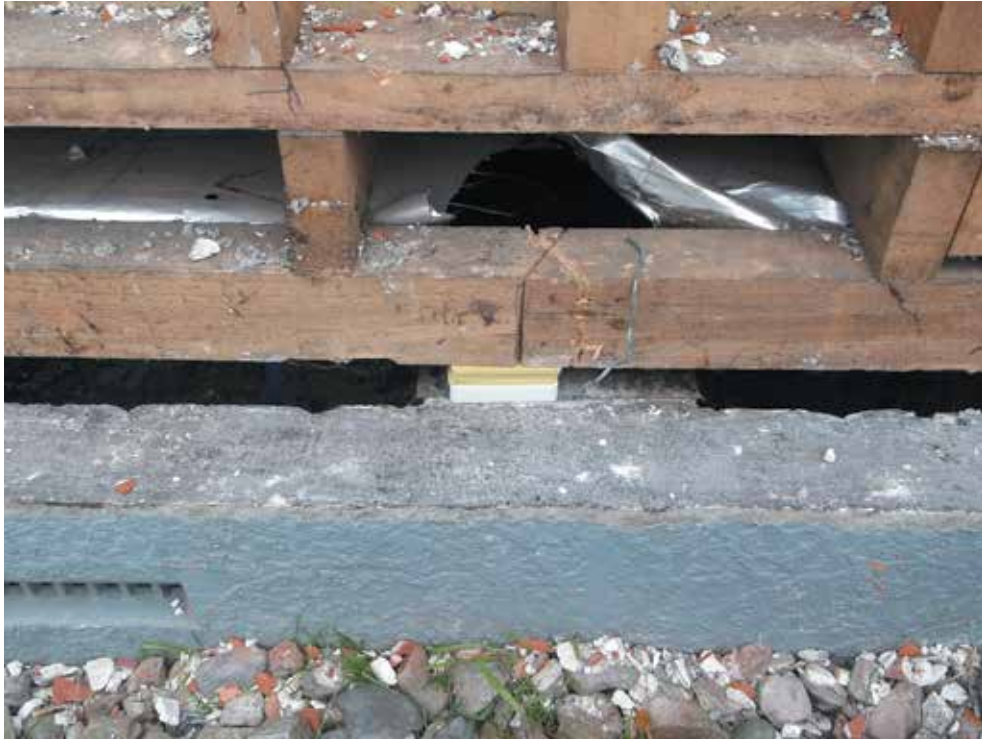
Image 5: New bearer packed for superstructure releveling (still to be wired down)
