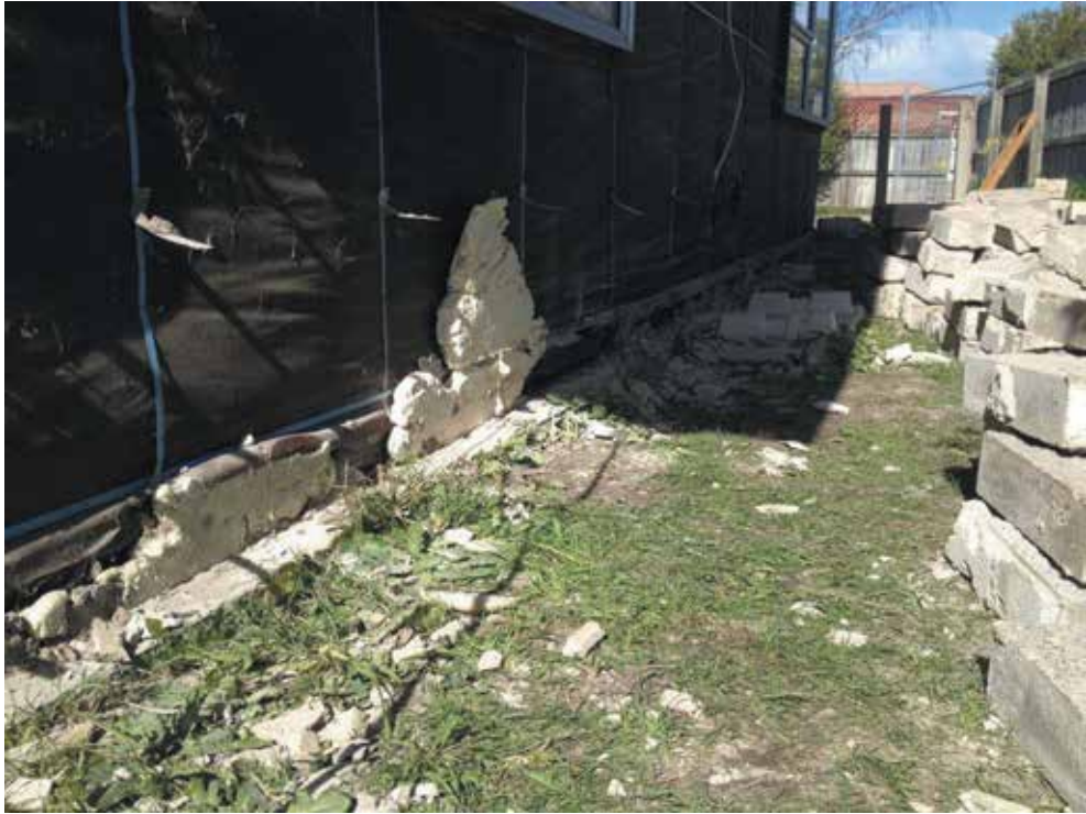
Image 12: Resin intrusion into cavity
