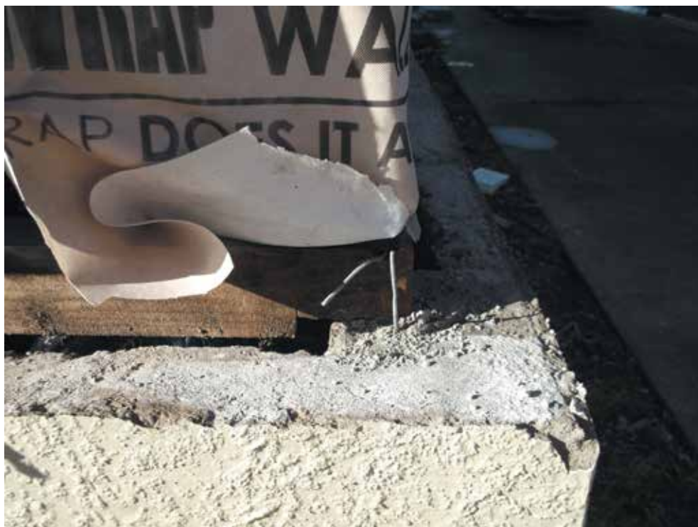
Image 6: Bearers notched where required to avoid maximum packing at other support positions
