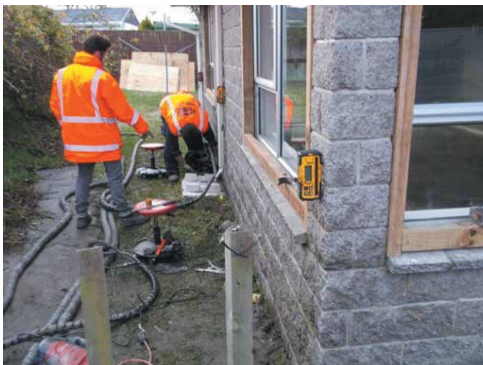
Image 7: Resin injected to return dwelling to level
