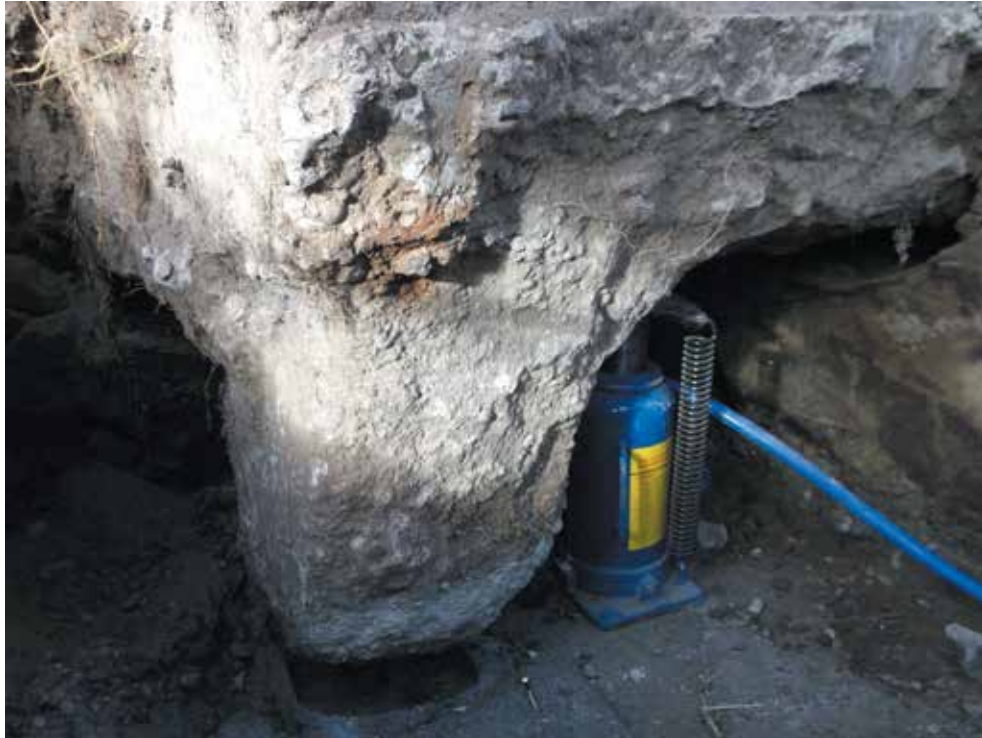
Image 7: Jacks in place. All points of foundation lifted simultaneously
