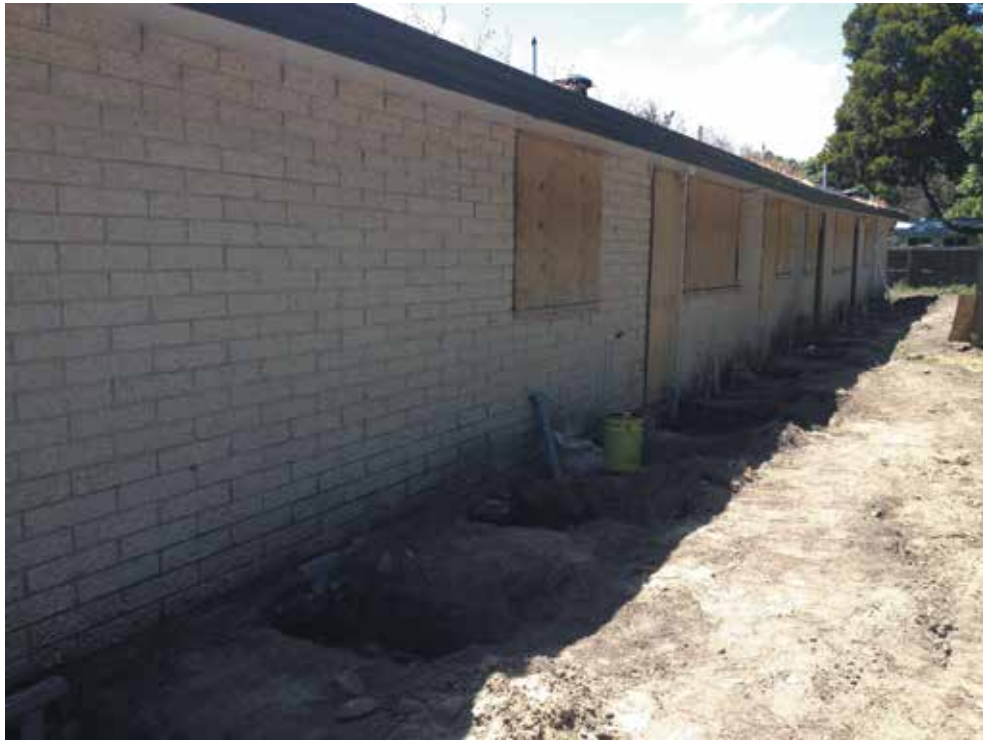
Image 5: Screw piles in place with brackets attached to foundation perimeter beam
