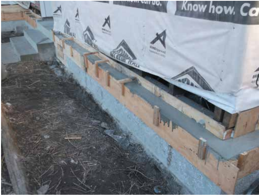
Image 9: Cementitious grout poured into formwork that was preset to correct level
