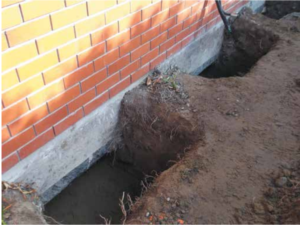
Image 4: Jacking points excavated as per engineer's design
