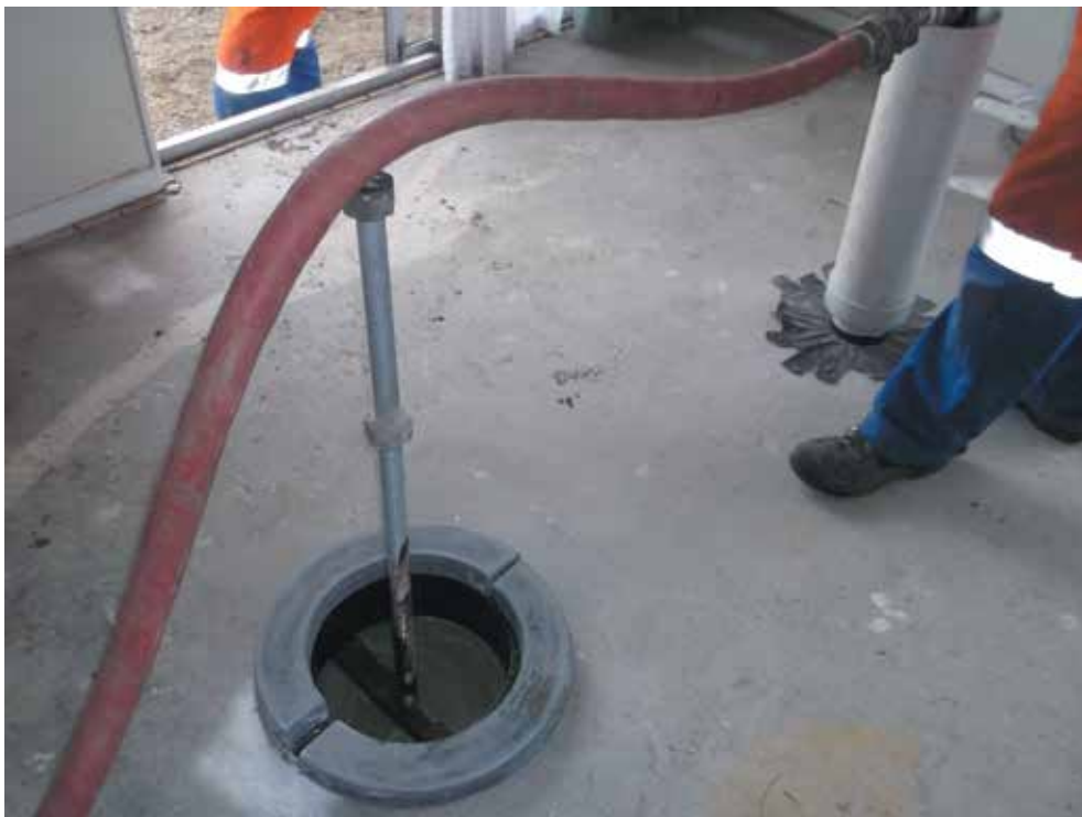
Image 8: Concrete slab lifted at same time as foundation. Void fill poured
