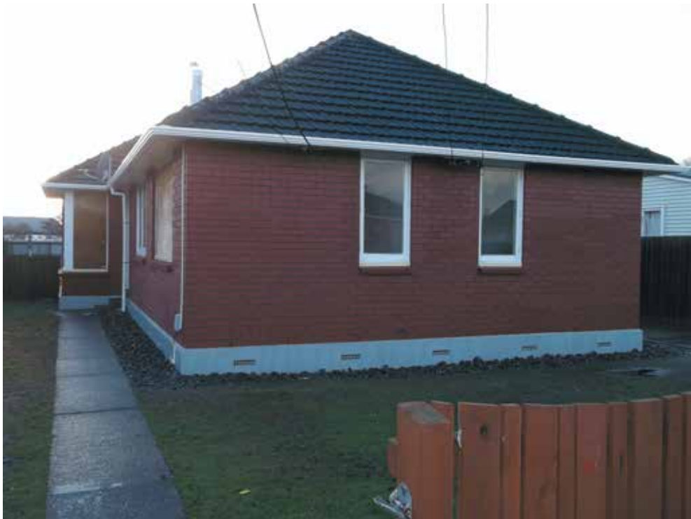
Image 10: Repairs complete. New veneer cladding with replastered foundation
