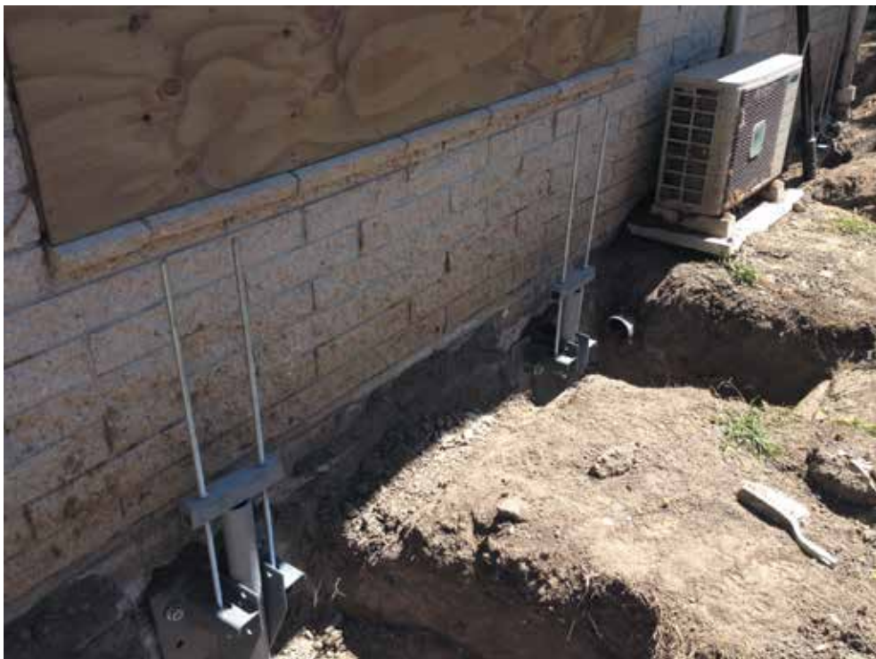
Image 6: Lifting brackets attached to foundation and screw piles
