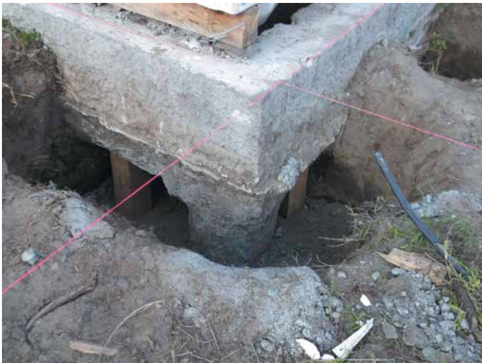
Image 8: H5 timber packers installed before jacks removed
