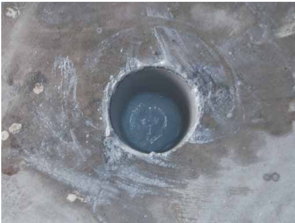
Image 9: Void filled under internal slab making sure DPM of slab maintained
