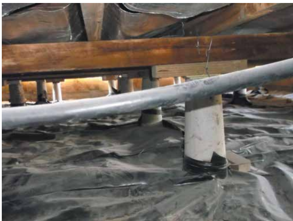
Image 7: Subfloor jacked and packed
