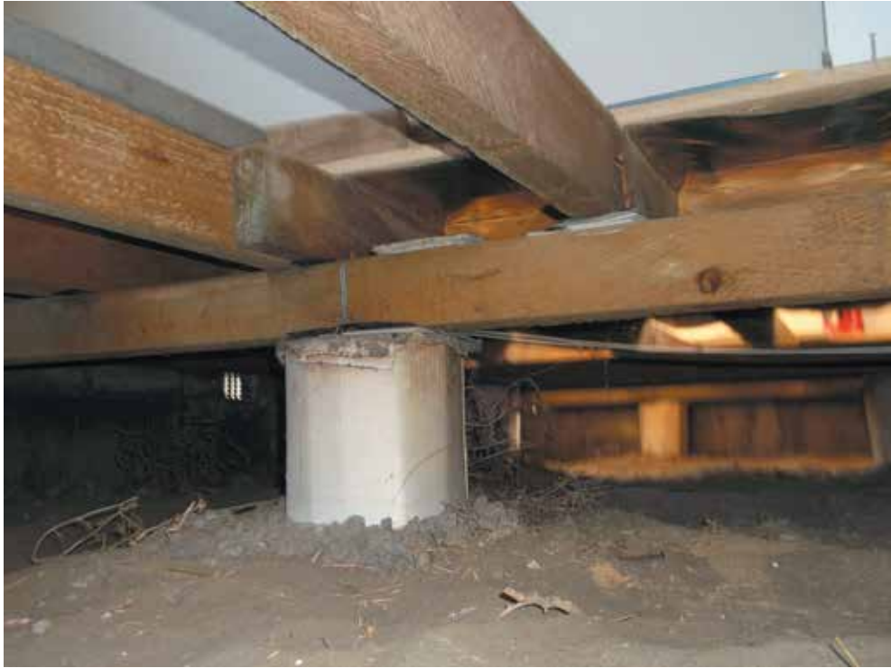
Image 6: Individual joists packed if required to level localised areas
