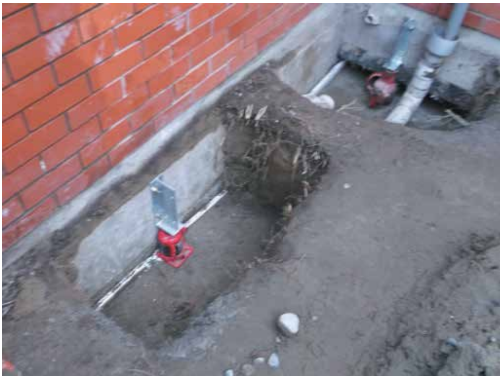
Image 5: Jacking pads poured and brackets installed ready for lifting
