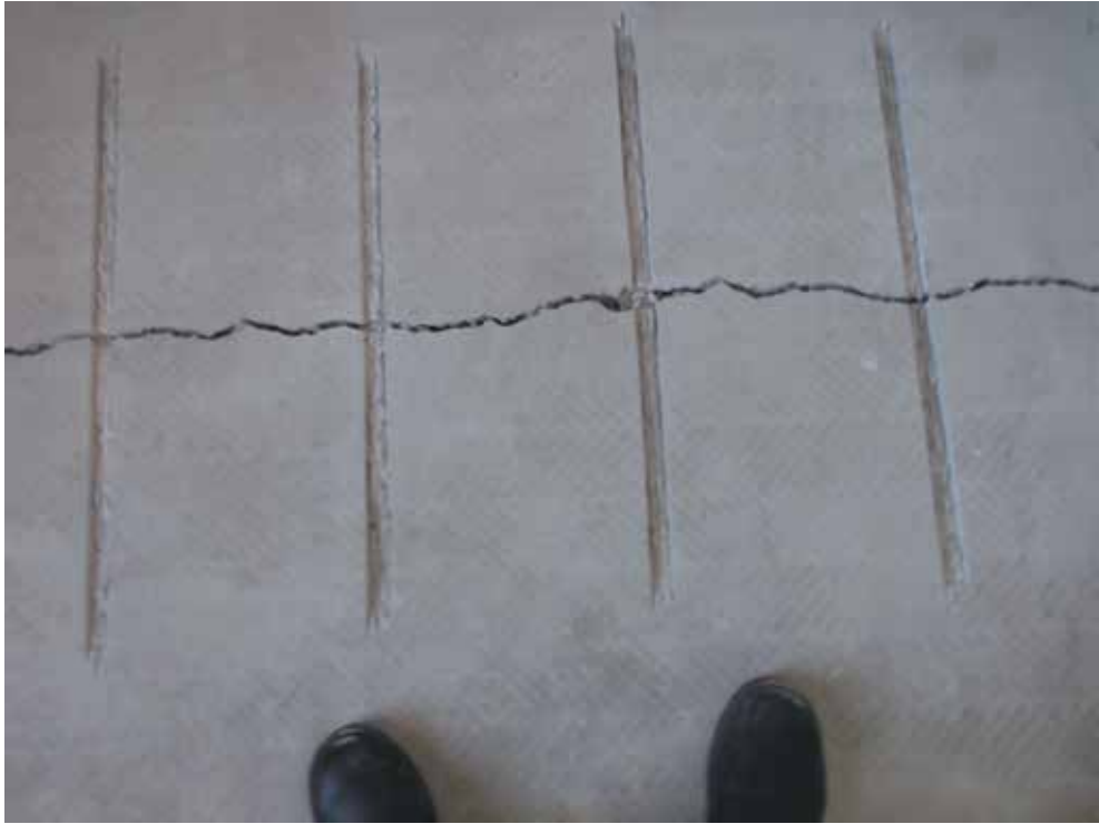
Image 10: Channels cut into slab perpendicular to crack
