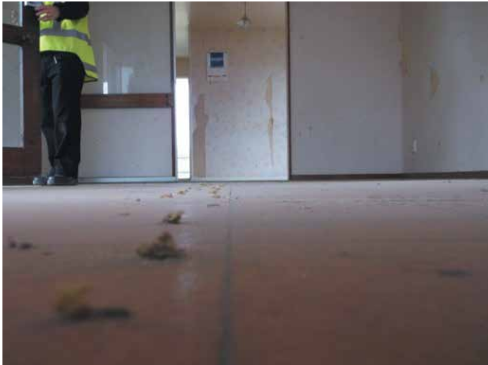
Image 11: Floor reinstated to level
