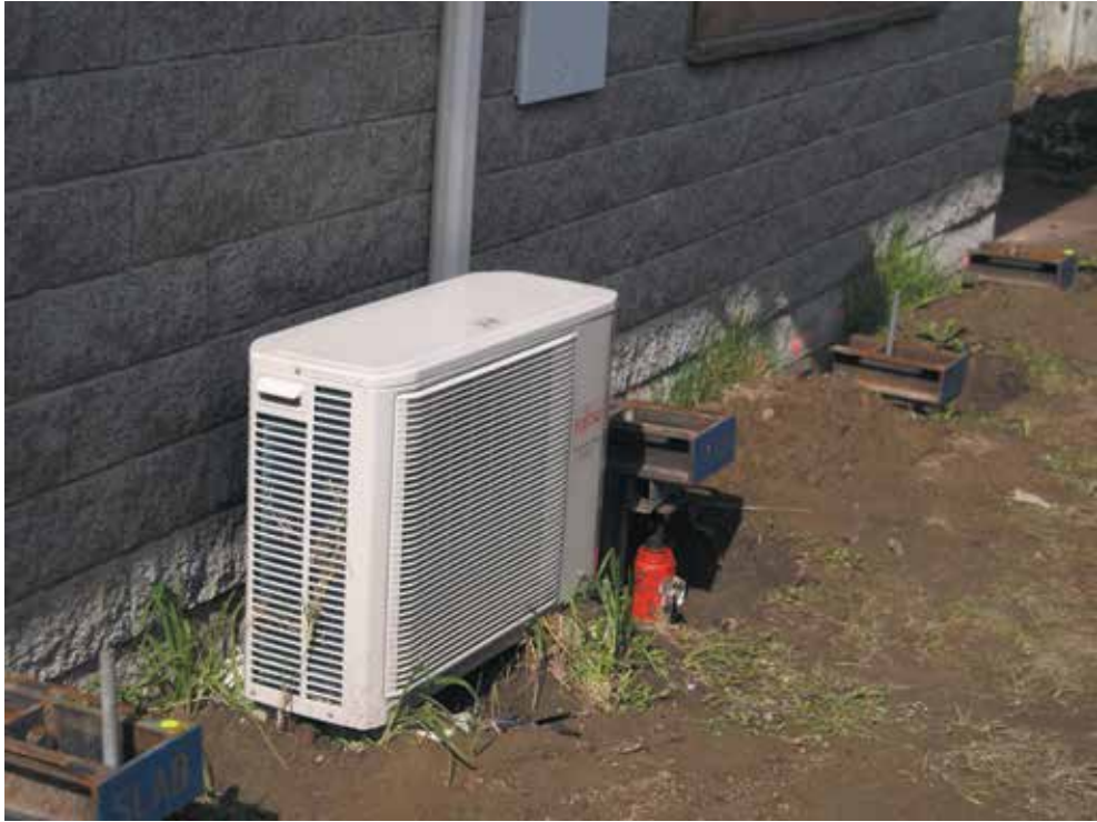
Image 7: Lifting brackets and jacks installed for foundation lift
