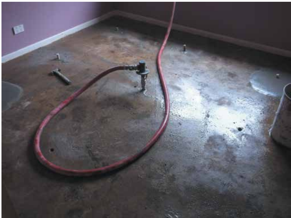
Image 8: Void filling epoxy levelling compound injection points
