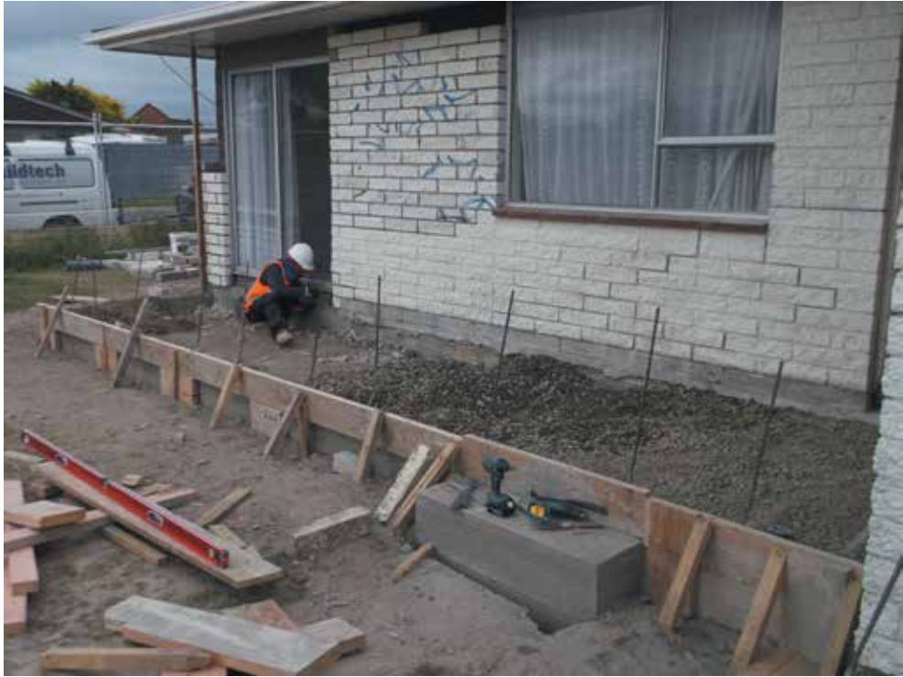
Image 11: Mortar repointed and patios being reinstated
