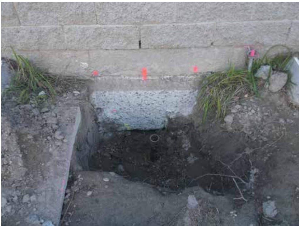
Image 6: Screw piles installed at depths determined by geotechnical ground conditions
