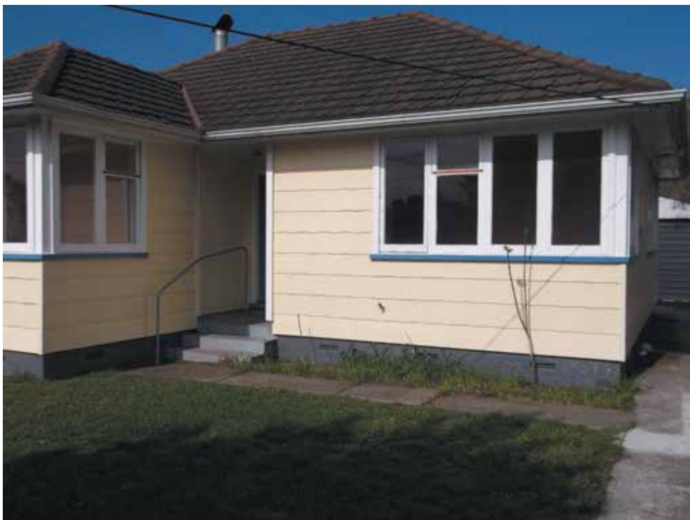
Image 7: Fibre cement sheet replaced bottom row of asbestos weathersiding
