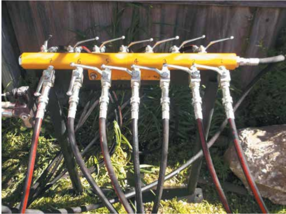
Image 7: Mechanical jacking manifold system
