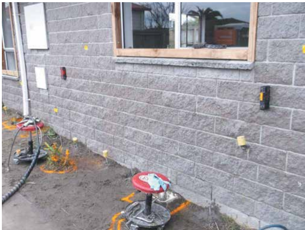
Image 6: Resin injection tubes inserted at specified centres
