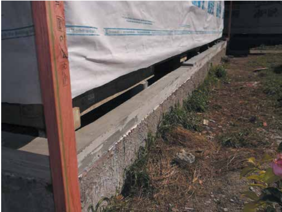
Image 10: Foundation topping poured and formwork removed
