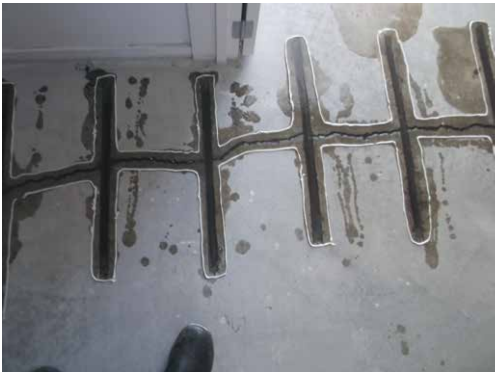
Image 11: Reinforcing bars inserted and epoxy compound put in place (see Figure 1)
