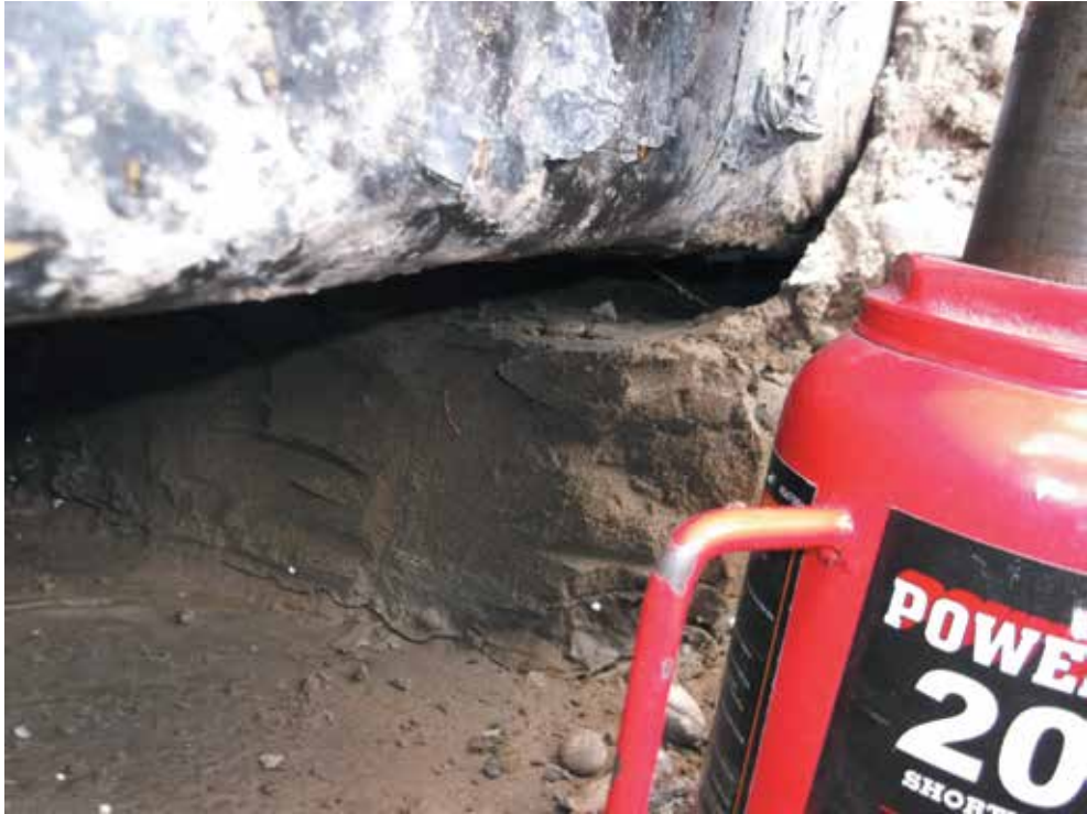
Image 7: Exterior foundation jacked to required level
