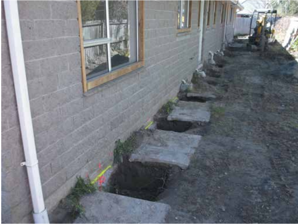
Image 5: Jacking points excavated at centres determined by structural engineer
