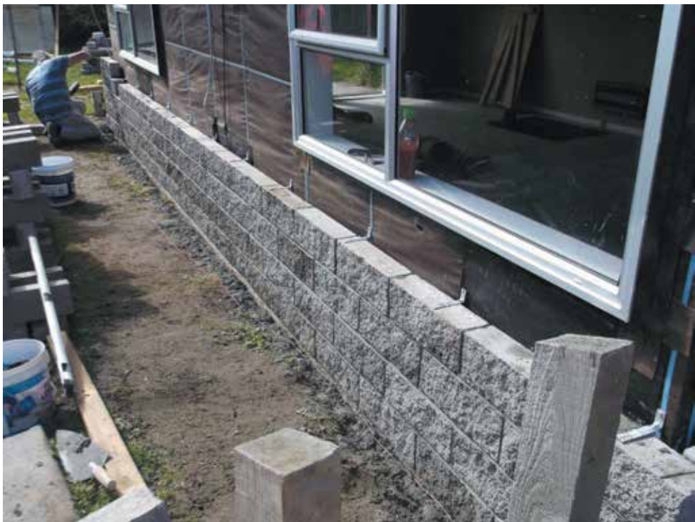
Image 13: Affected area reclad
