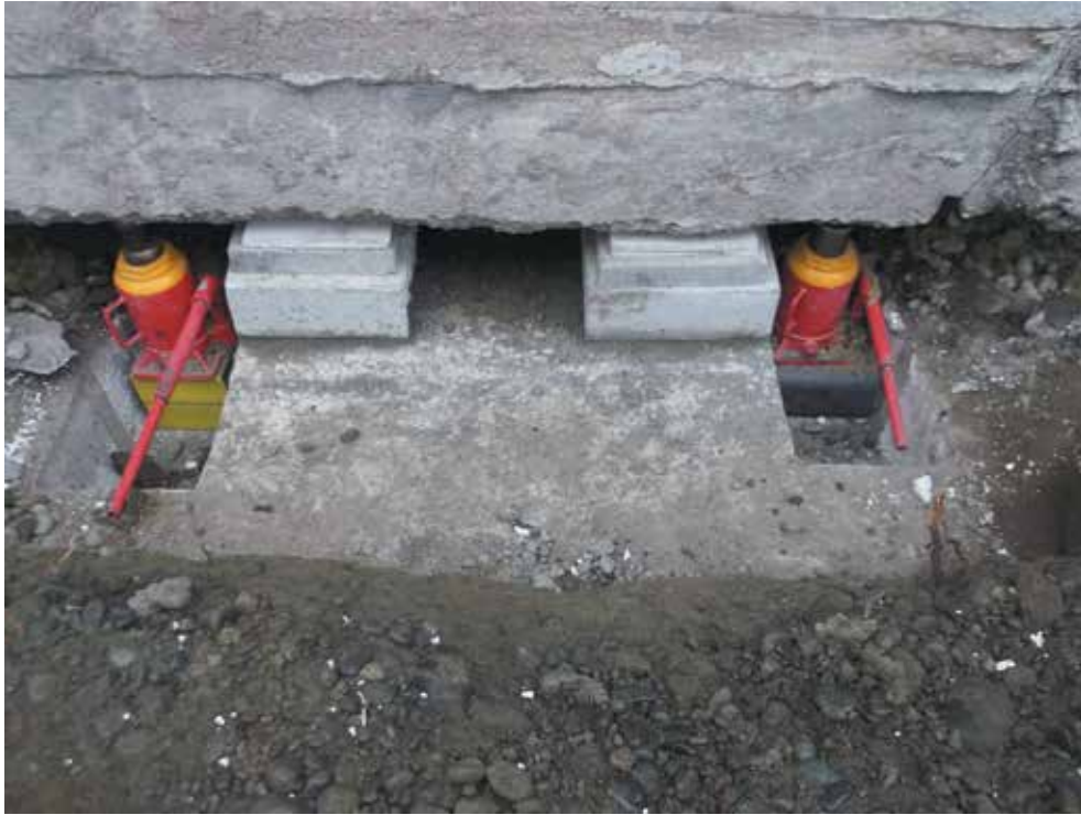
Image 7: Jacked and supported foundation
