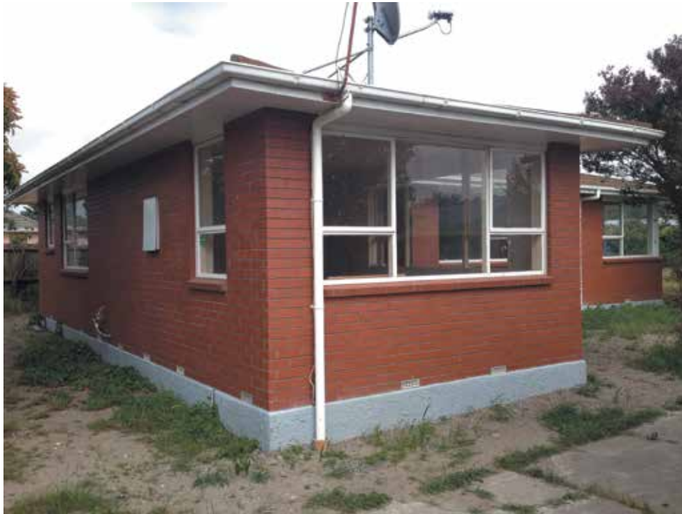
Image 11: Foundaton repaired and house reclad
